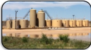
LMS Water Treatment Plant
