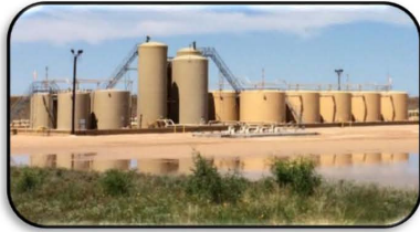
LMS Water Treatment Plant
